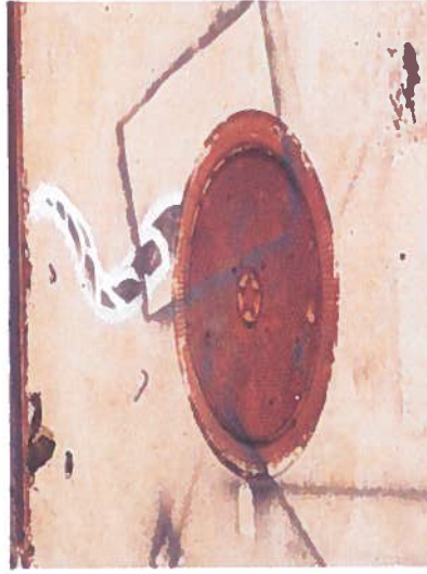
FIGURE 21: Several different styles of manhole cover are seen on the south side of the Boiler Shop. Further investigation is required to determine if these are interconnected or serve separate facilities such as sanitary sewer or industrial waste.
