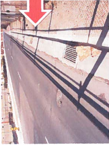
FIGURE 25: Another view of the public storm inlet in the east curb line of Second Street SW as viewed from the south looking north with a second inlet located upstream.
